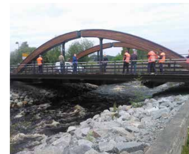
Photo 9. Finnish experts learning about wooden bridges in Norway in summer 2014. (Photo: MEE)
