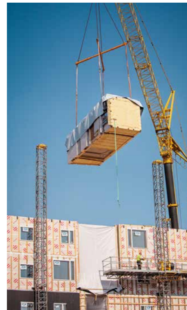
Photo 8. Prefabricated CLT modular units being set up. (Photo: Puuinfo Oy)
