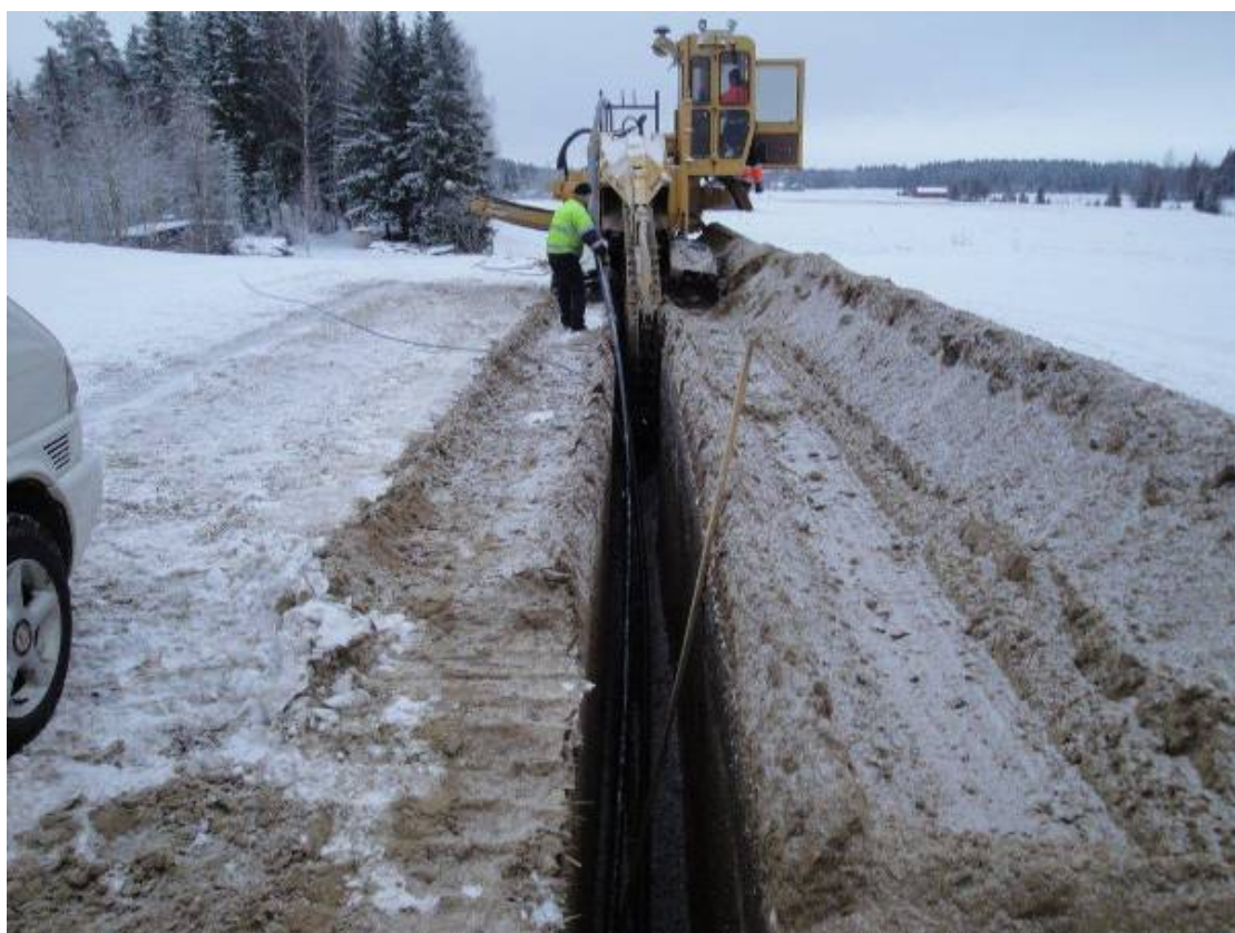
A cable trench made using a trencher - winter 2010 (Photo: Reiniko Oy)
