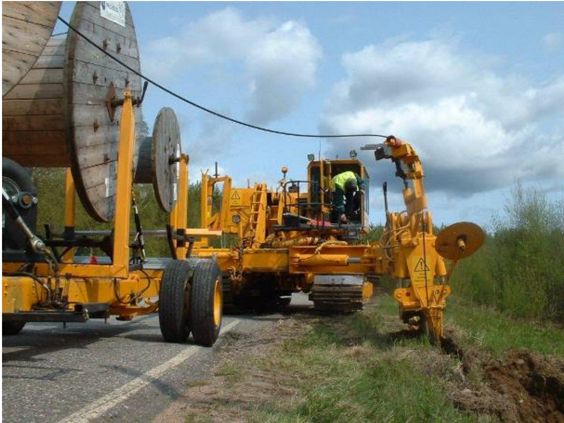
Cable ploughing carried out as a separate project (Photo: Reiniko Oy)
